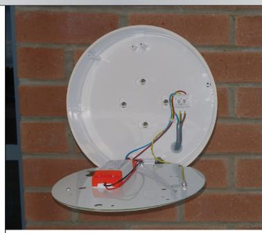
STEP 3 Fix base to mounting surface
