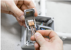
Place the wired connector in the Gelbox.
