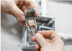
Place the wired connector in the Gelbox.
