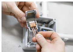
Place the wired connector in the Gelbox.
