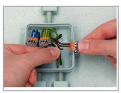
Termination: Insert stripped solid conductor until it hits backstop.
