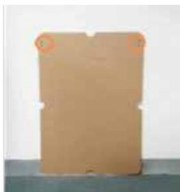
Use the positioning cardboard to draw screw hole positions on the wall
