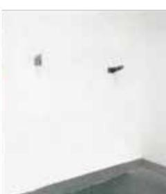
Attach the fixings using the M6 bolts, Torque at 6NM. (Floor installation)
