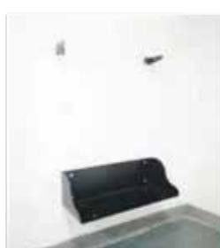
Install the battery bracket with M6 expansion bolts (Wall installation)
