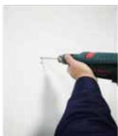
Drill 4 holes, hole depth greater than 70mm for expansion bolts.
